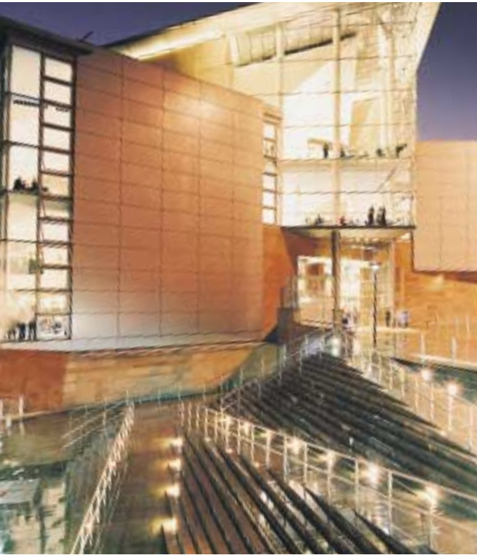
Natural Stone, Bridgewater Hall, Manchester
