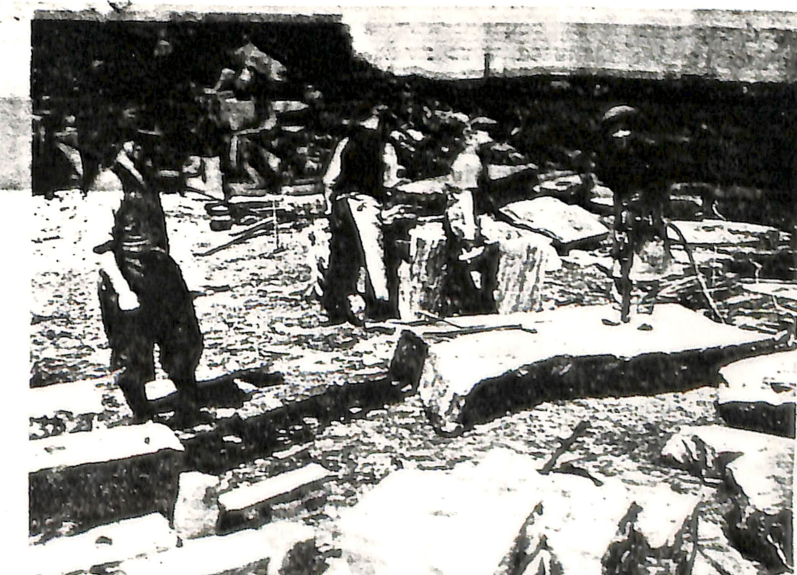
Trimming Paving Stones.
