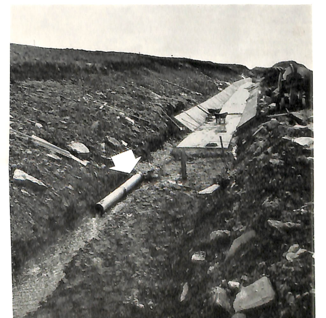
Typical ditch showing preparatory drainage (arrowed) prior to flagging main channels.
