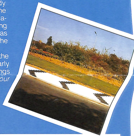
Very visible chevron markings in concrete block paving allow for forward visibility — and low maintenance costs.
