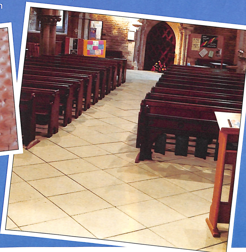
(Above) Warm water pipes are coiled over base plates, followed by a screed. (Right) The Charnwood pavings are bonded directly to the screed.
