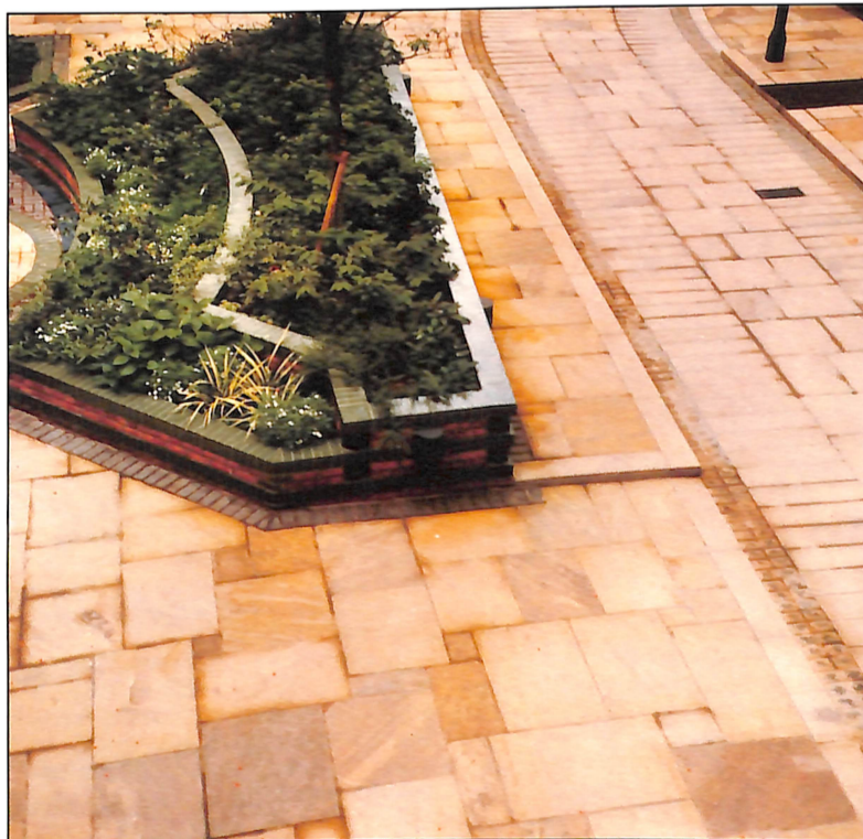
A mixture of random size riven pavings and sawn pavings was used for the courtyard of St. James's Court Hotel in London.
