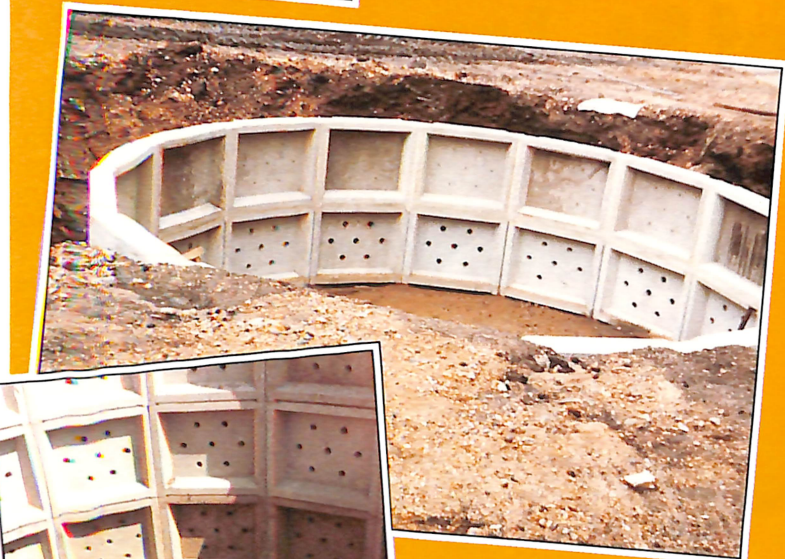
Lifting equipment is needed for the segments of the 6 metre diameter soakaway. (Top) Non-perforated segments are used above the level of the inlet pipe. (Left) Soakaways seven metres in depth are not exceptional.
