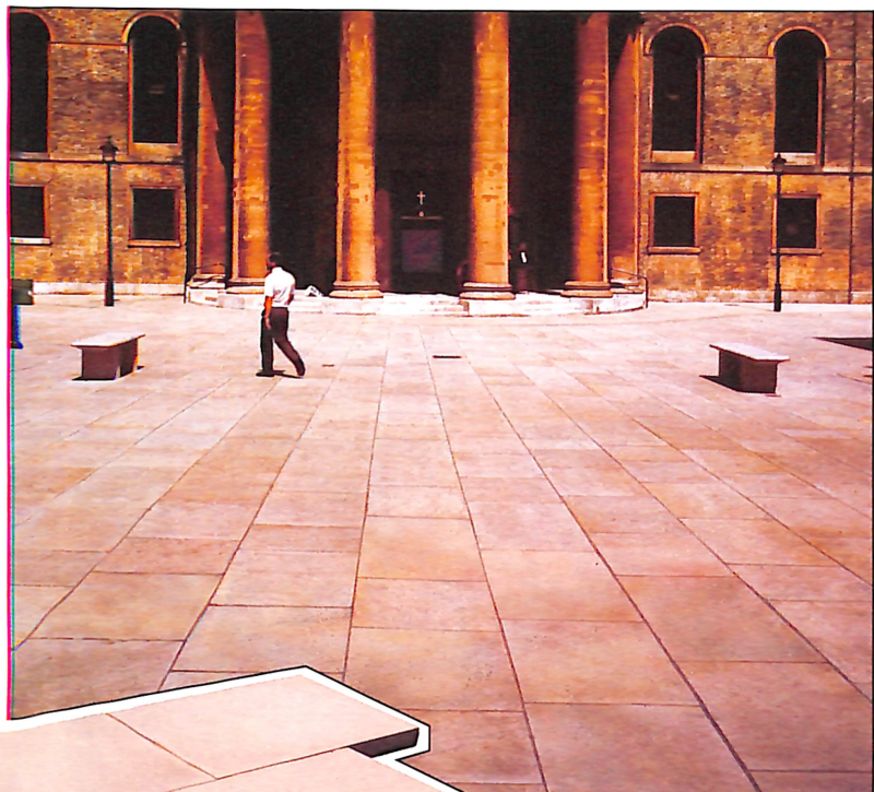
Fine-sawn natural York stone pavings, here in Wyndham Place, London, are widely used on prestige projects.
