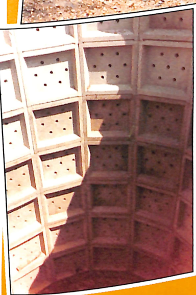
Lifting equipment is needed for the segments of the 6 metre diameter soakaway. (Top) Non-perforated segments are used above the level of the inlet pipe. (Left) Soakaways seven metres in depth are not exceptional.
