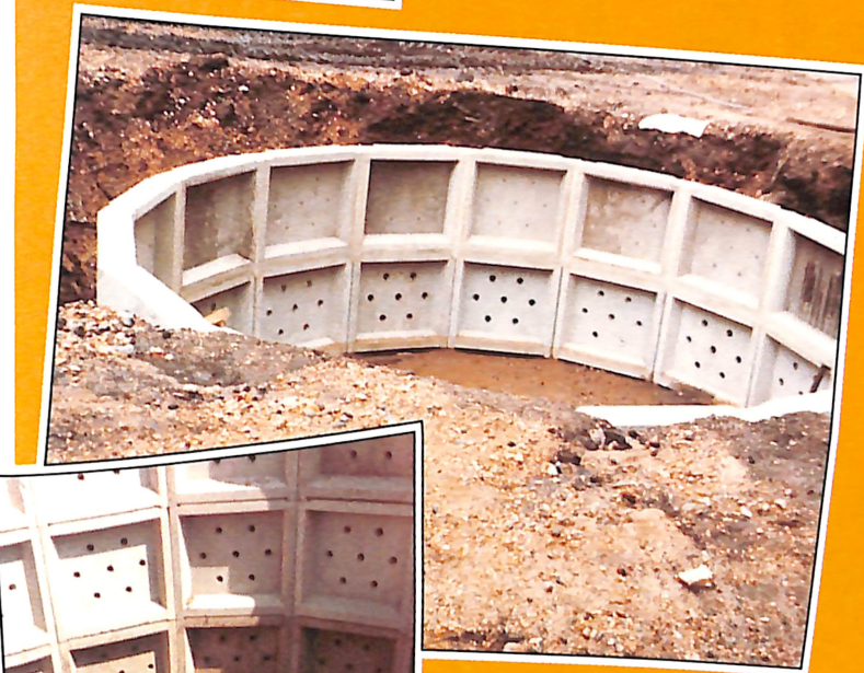
Lifting equipment is needed for the segments of the 6 metre diameter soakaway. (Top) Non-perforated segments are used above the level of the inlet pipe. (Left) Soakaways seven metres in depth are not exceptional.
