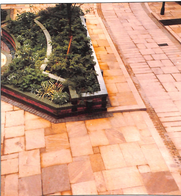
A mixture of random size riven pavings and sawn pavings was used for the courtyard of St. James's Court Hotel in London.
