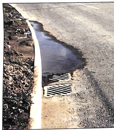
This is typical of the ponding which often occurs at low spots with conventional drainage. It is not possible with the Beany Block because there are elliptical drainage inlet openings at half metre intervals.
