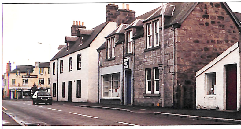
(Below) The footway could not be raised because of steps and house d.p.c.'s but that did not prevent resurfacing of the carriageway. Alternate Beany Blocks were reversed to drain both carriageway and footway.
