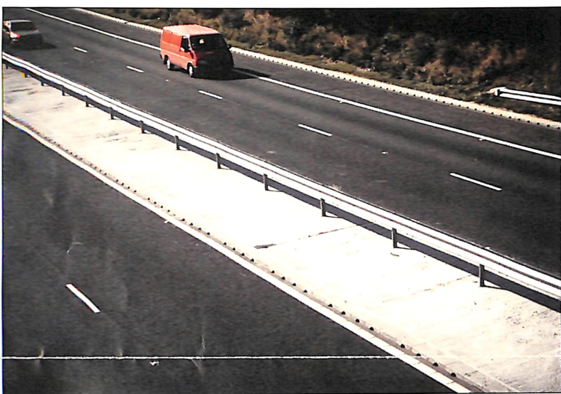
(Above) Every fifth Beany Block along the central reserve has been reversed to take water from the carriageway and the reserve.
