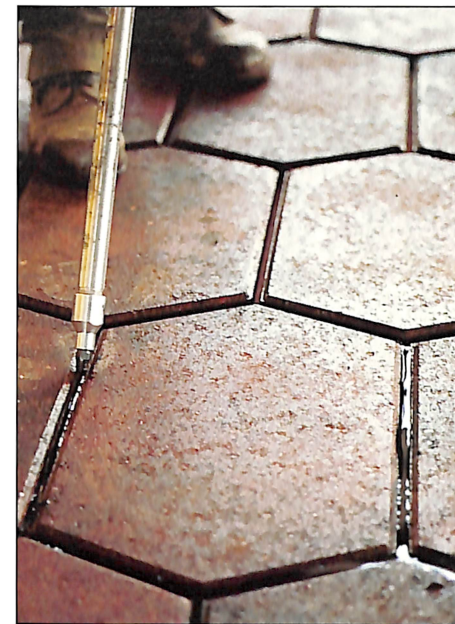
Applying the joint sealant to Petrapave.
