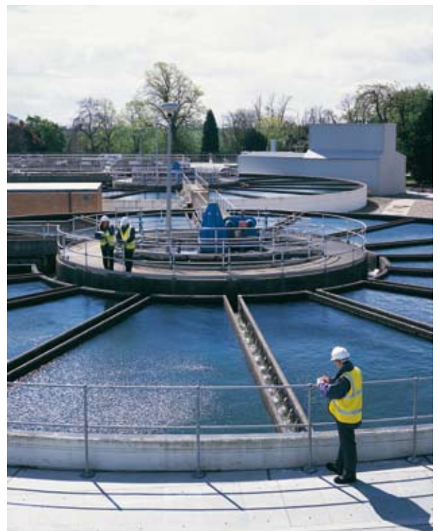
Broken Scar water treatment works, Darlington. Drinking water inspector checking clarifier performance
