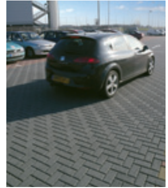
Permeable Paving Sustainable Urban Drainage systems with a permeable surface for effective water management.
