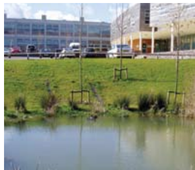
Hazeley School, Milton Keynes. Concrete block permeable paving in car parks treats water feeding wildlife ponds and elsewhere is used for water harvesting for toilet flushing.
