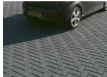
Permeable Paving Sustainable Urban Drainage systems with a permeable surface and calibrated sub-base for effective water management.
