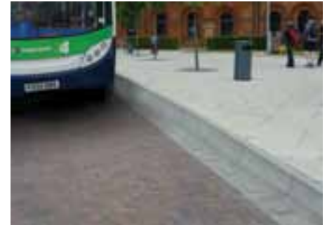
Bus Stop Kerb Variable height kerb systems to suit different public transport entry levels.
