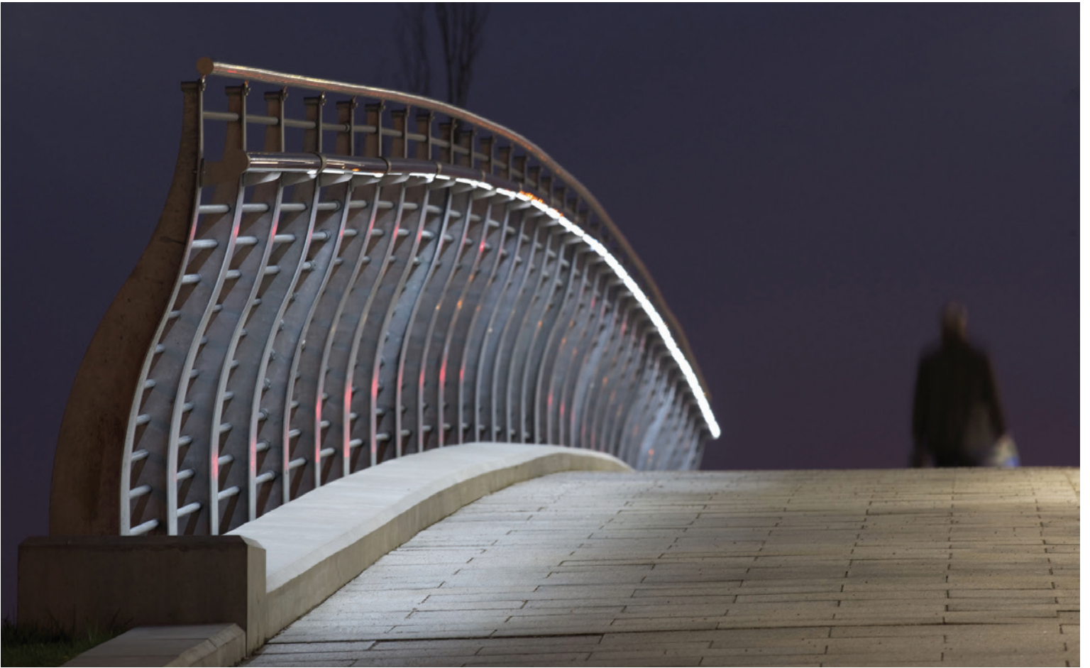
LED luminated handrails
