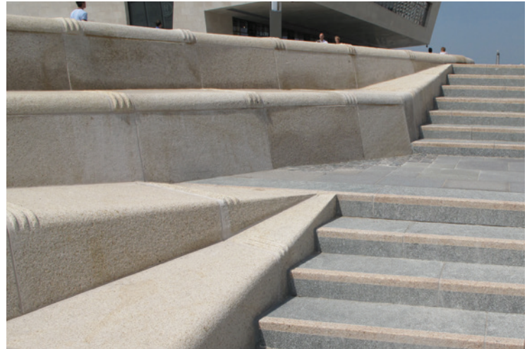
Steps with inserts, cladding, coping and solid wall units, Pier Head Liverpool
