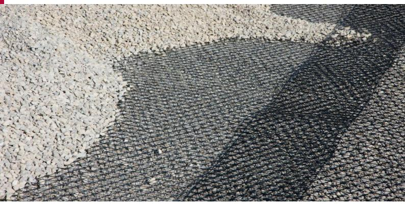
A special grade of GeoGrid that has been developed with the UK's market-leading grid supplier, Marshalls MG15 Grid provides additional stability within the sub-base of a Priora permeable pavement.
