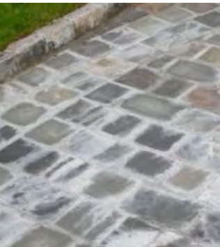
Cement staining on setts
