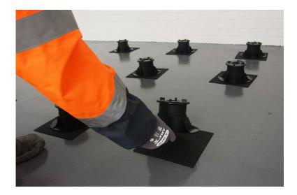
Roughly lay out sufficient pedestals for 4 or 5 paving units. When laying out, consider moving the centre line to minimise cutting around the edge and ensure full units are employed. This is ideal for areas of high foot traffic (eg: door openings).
