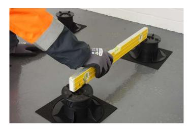
Lay the paving units, ensuring the pedestals are place in the correct formation to fully support the unit. For the correct number of pedestals for each plan size, see diagram below:
