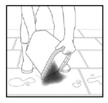
Open the tub and cut open the vacuum bag. Empty the joint compound material onto the paving surface and start to brush into the joints. Continuously keep the paving area saturated with water and so the area doesn't dry out
