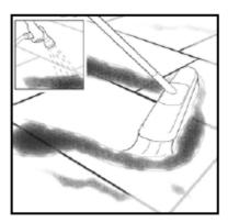
Brush the jointing material into the joint areas with plenty of water to allow it to flow into the joints easily. Brush material diagonally (45°) to the joint. Ensure that the joint void is completely full. The jointing material must be used within one hour of opening the vacuum pack.
