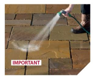
Whether you are laying Weatherpoint 365 in the rain or dry, always thoroughly saturate the paved area with a hose or watering can and leave for 10 minutes to absorb. Re-saturate before applying Weatherpoint 365. Failure to wet the paving could temporarily stain the paving's surface.
