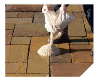
Open the tub and cut open the vacuum bag. Empty the Weatherpoint 365 material onto the paving surface.
