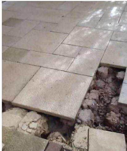
Spot bedding giving poor support
