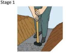
Dig a trench to the depth of a full block plus 150mm for foundation material. The width should be minimum of 2 times the wall thickness and the foundation material should extend 85mm to the front and rear of first course block.
