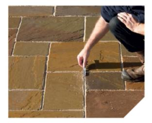
Sweep off any excess Weatherpoint 365 and store (see detailed instructions on tub). Strike off the joint using a standard brick jointer, top up any sagging joints with more Weatherpoint 365 and strike off again.
