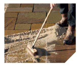
Brush Weatherpoint 365 material into the joint areas with a stiff sweeping brush, occasionally hosing with water to allow Weatherpoint 365 to flow into joints. Ensure that the joint void is completely full.
