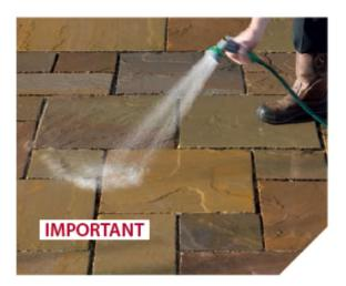
Whether you are laying Weatherpoint 365 in the rain or dry, always thoroughly saturate the paved area with a hose or watering can and leave for 10 minutes to absorb. Re-saturate before applying Weatherpoint 365. Failure to wet the paving could temporarily stain the paving's surface.
