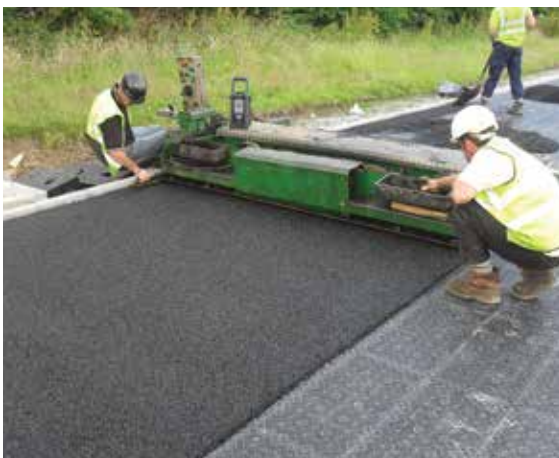
Figure 20.10 Construction of sports drainage and attenuation layer below school sports pitch in Hull (courtesy Phil Tomlinson)
