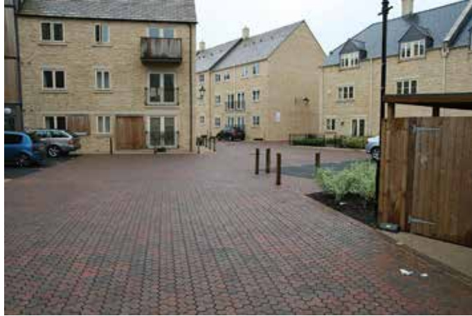
Figure 20.20 Concrete block permeable paving after a 50 mm rainfall event (courtesy EPG Limited)
