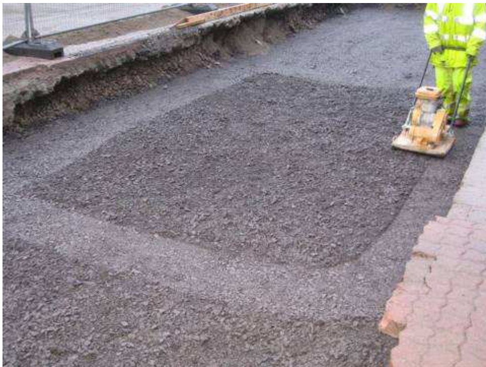
Figure 8. 150mm thickness of compacted Capping Material was installed throughout the test zone prior to installing polythene tanking.
