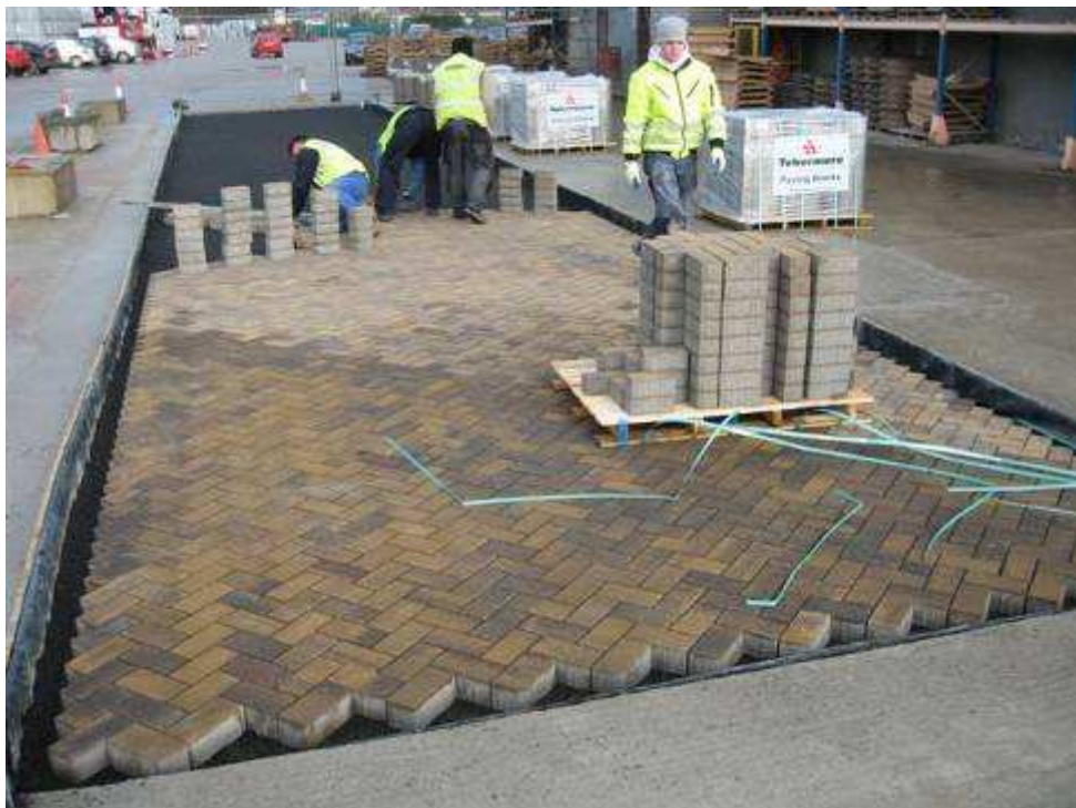
Figure 12. Permeable pavers were installed to a 45° herringbone pattern.
