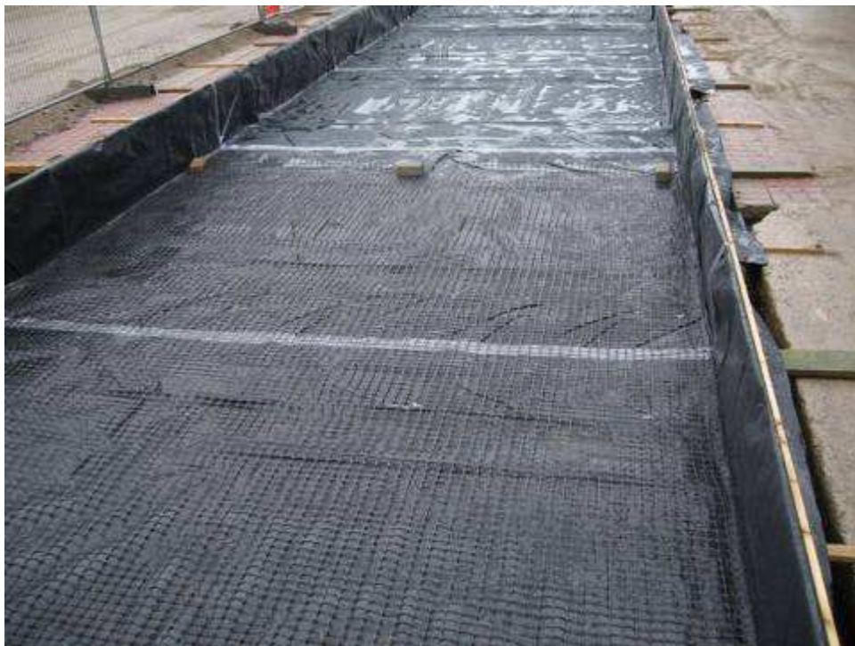
Figure 10. Test Item 4 required the installation of two layers of a geogrid material known as Tensor SS40. The lower layer is shown here directly over the polythene membrane.
