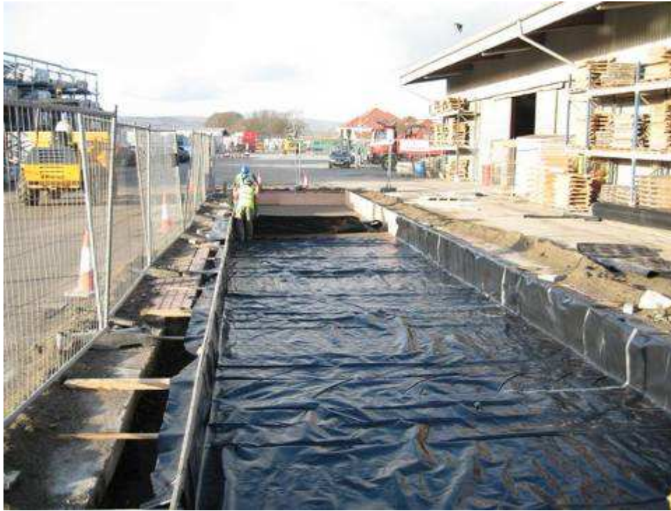
Figure 9. 2000 gauge polythene was installed to achieve tanked conditions for each Test Item.
