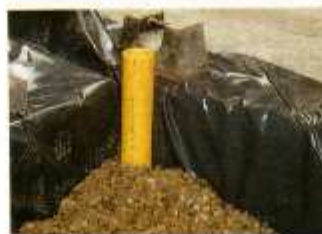
Fig 3. Vertical drains installed at each end of NUROLF allow the level of stored water to be measured.
