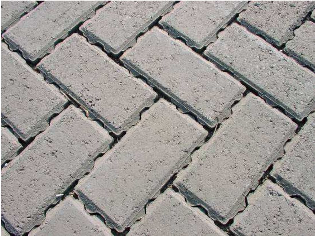
Marshalls Priora permeable pavers installed in herringbone pattern
