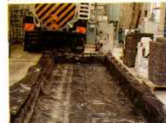
Fig 1. MURDOFF test site showing waterproof material prior to installation of crushed rock open graded roadbase.
