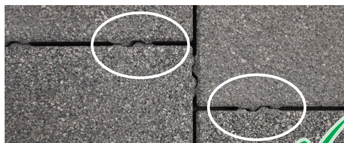
Correctly interlocking nibs
