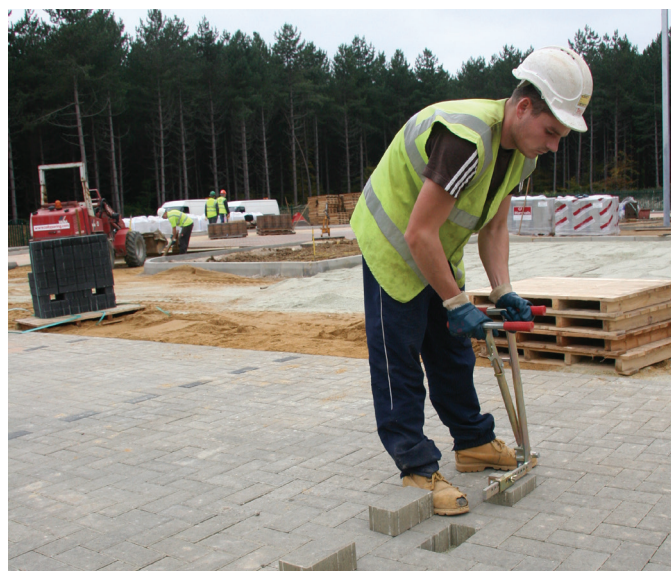
Manual block lifter in action
