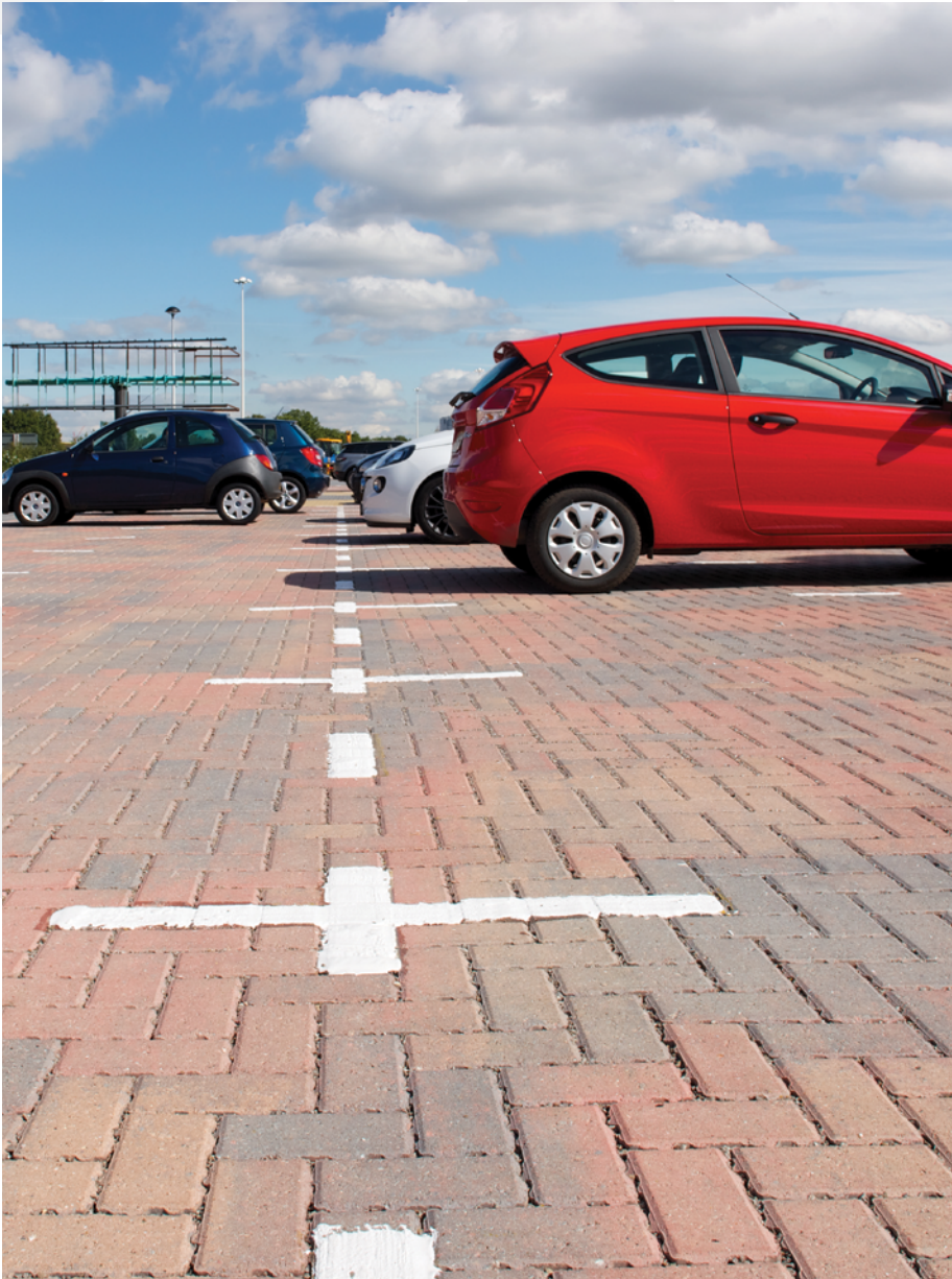
The nibs around the edge of each Piora block create voids so water can fall through into the sub-base
