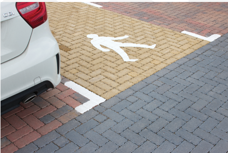
Colour can be used to differentiate parking bays
