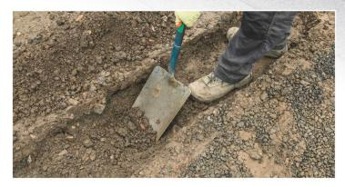
1. Excavate a suitable concrete strip footing, normally 100mm lean mix, to support the Driveline Drain units, outfall and Rodding Boxes.
