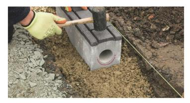
3. Before installing the Driveline Drain units apply a 5mm bead of adhesive around the bottom half of the drainage hole avoiding the top of the aperture. Lay the units onto a freshly mixed workable concrete bed, making sure you achieve a tight connection between each unit.
