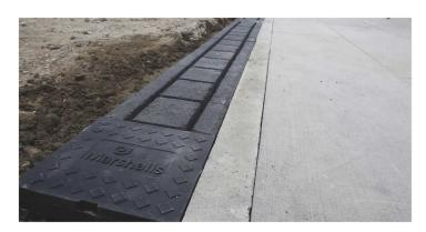
5. On a flexible install lay the paving 3-5mm above the Driveline Drain units. On a rigid install lay the paving flush to the Driveline Drain units.
