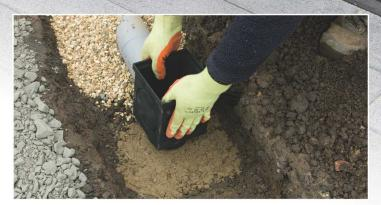
2. Driveline Drain outfalls and Rodding Boxes should be installed first along with relevant pipe work to existing underground pipework, soakaway or SuDs compliant system\*.
