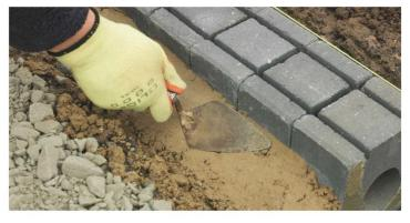
4. Haunch the units using bedding concrete of an appropriate thickness and depth.
