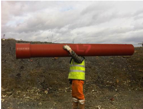
Figure 3. DN300 Brand 1 pipe lifted by one man at shoulder level.
