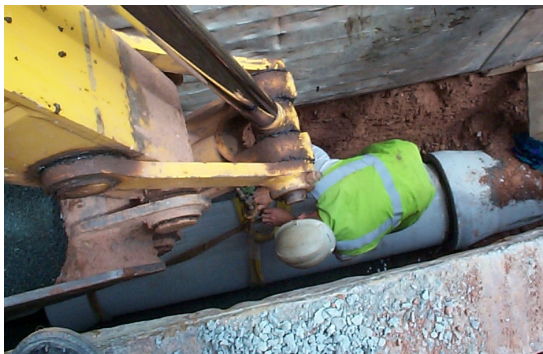
Pulling the pipe home with a strap
