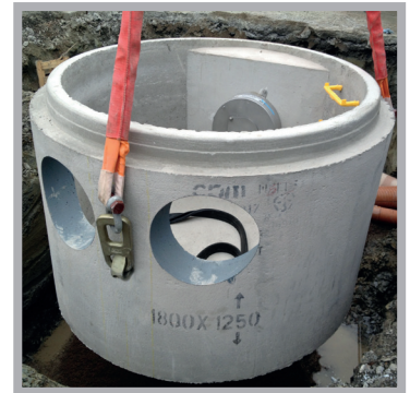
1800mm sealed chamber complete with Optimum Hydro-Brake®
