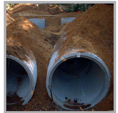
End entry manholes
