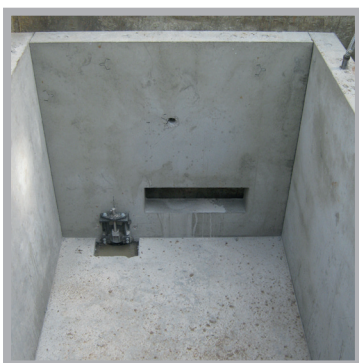
Once-piece chamber with inlet and outlet holes
