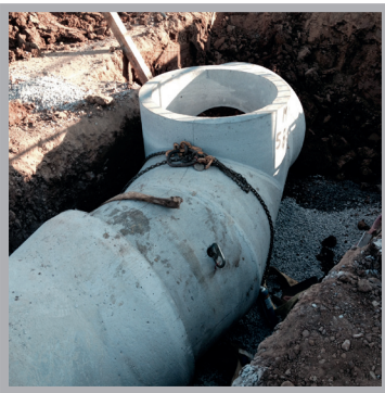
900mm off 900mm mid entry manhole
