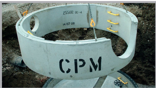
2550mm sectional installation, upper ring with half formed hole for 900mm pipe and formed inlet hole
