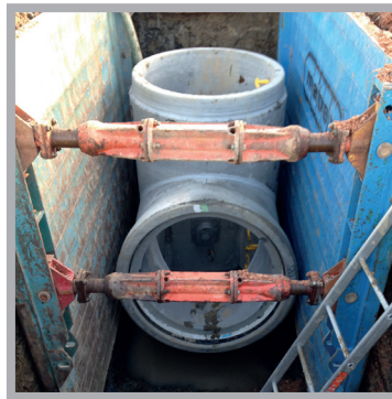
1200mm end entry manhole complete with hydrobrake
