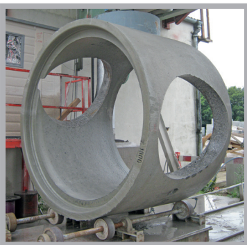
1800m sealed manhole being cored for a 900mm internal diameter pipe
