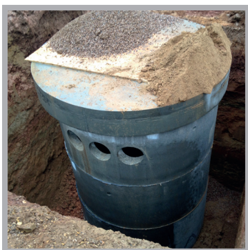
2100mm base chamber and section complete with pump pipework cut out in chamber wall
