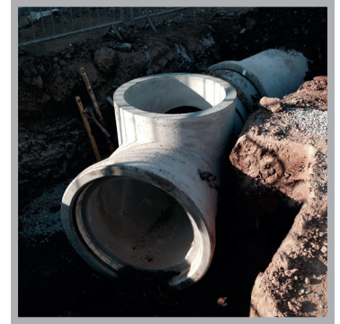
1200mm side entry run being installed
