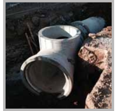
1200mm side entry run being installed
