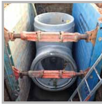
1200mm end entry manhole complete with hydrobrake
