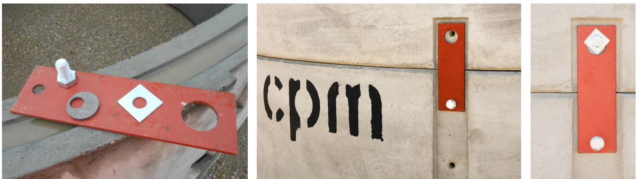
Fig A2 - Joint Connecting Plate
