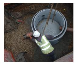
Once installed, the unit should be checked for level. The unit is backfilled with pipe bedding to 150mm over the pipes after which suitable backfill can be used unless the contract requires otherwise.
