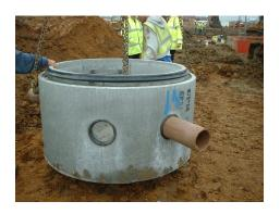
The unit with the butt pipe is jointed onto the pipeline.
