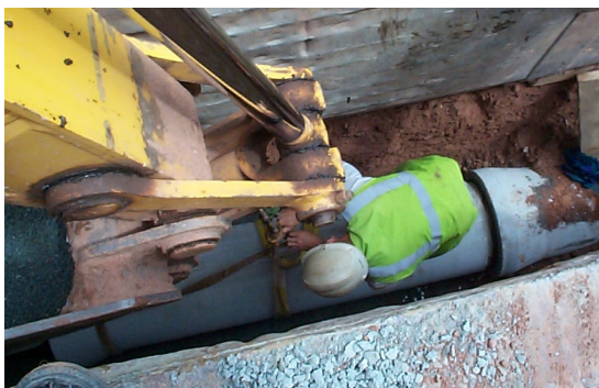
Pulling the pipe home with a strap
