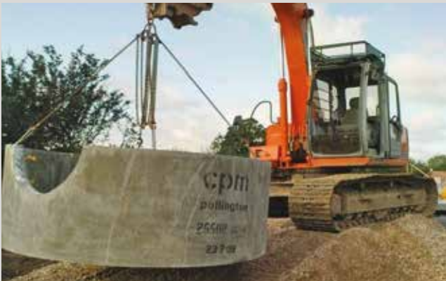
2550mm sectional installation, base chamber complete with half formed hole for 750mm pipe
