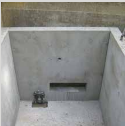
Once-piece chamber with inlet and outlet holes
