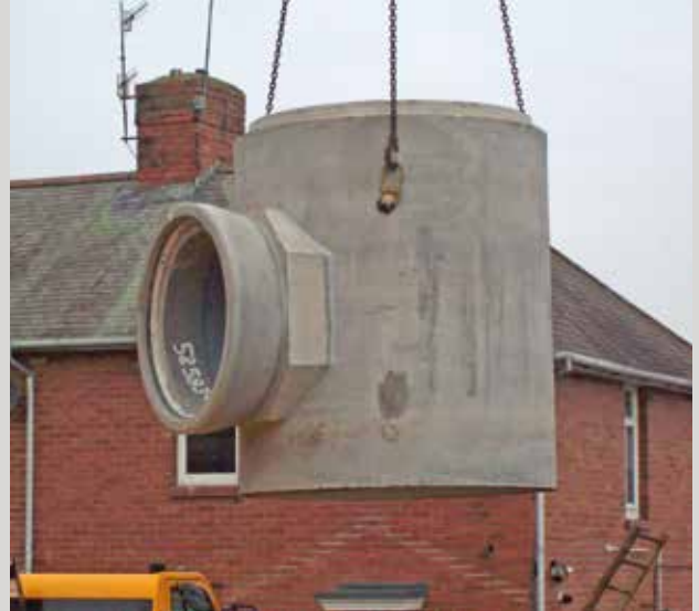
Single part 1800mm sealed manhole complete with pre-fitted 1200mm butt
