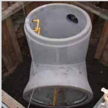
1350mm stop end bend complete with high level inlet
