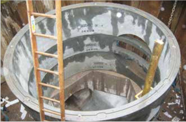
3000mm sectional chamber installation with a letter box opening for 1500mm concrete pipe
