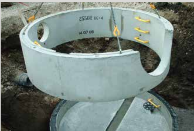
2550mm sectional installation, upper ring with half formed hole for 900mm pipe and formed inlet hole
