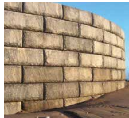
300mm wide strip of geogrid wrap through the blocks extending full length back in to reinforced fill zone
