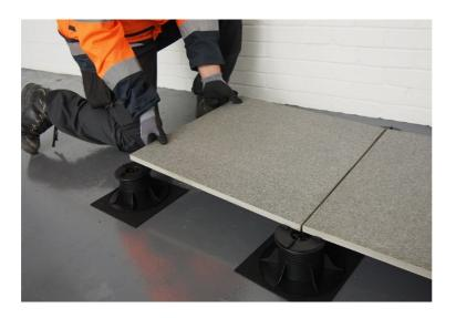
Use a spirit level to check finished level of the paving units. Use the MPAK Adjustment Key to make fine adjustments where required.
