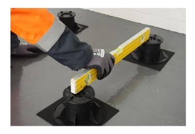
Lay the paving units, ensuring the pedestals are place in the correct formation to fully support the unit. For the correct number of pedestals for each plan size, see diagram below:
