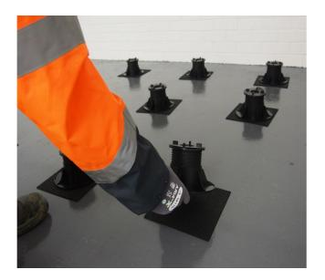
Roughly lay out sufficient pedestals for 4 or 5 paving units. When laying out, consider moving the centre line to minimise cutting around the edge and ensure full units are employed. This is ideal for areas of high foot traffic (eg: door openings).
