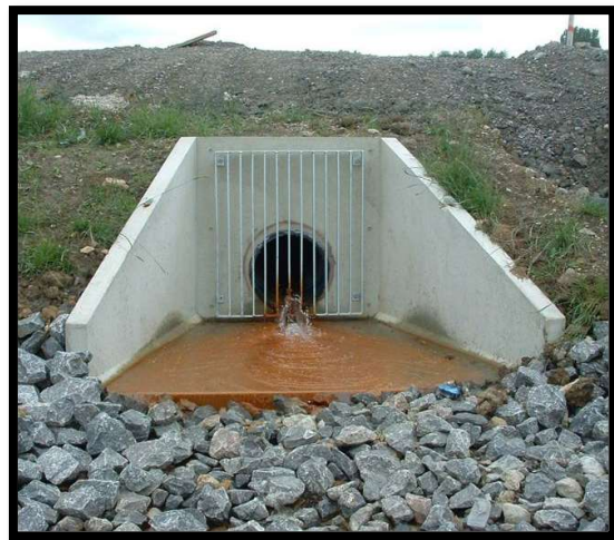
Fig 4 – Typical Marshalls Civils & Drainage Installed Outfall Headwall Unit
