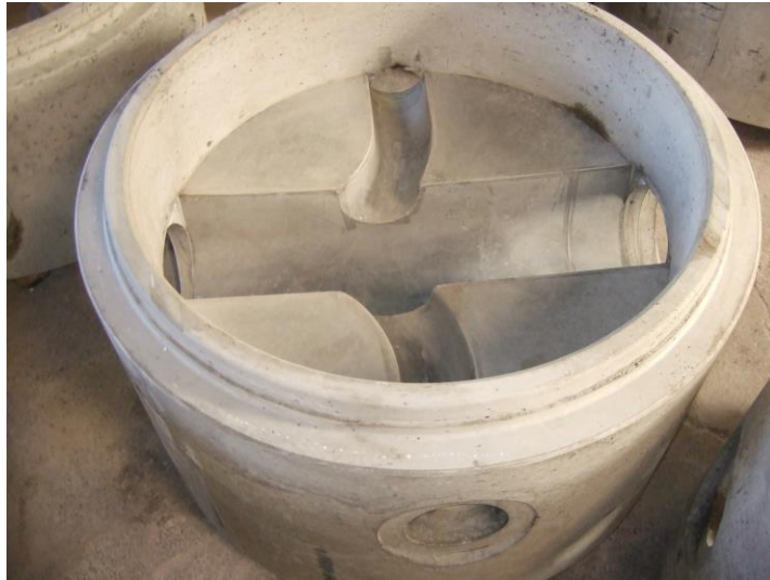
Typical MH base unit showing preformed benching
