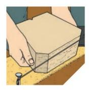
Place sub-base material (MOT Type 1 or similar) into the trench and compact. Spread a layer of sand, approximately 30mm, over the foundation material as this will make it easier to level first course block.
