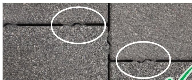
Correctly interlocking nibs
